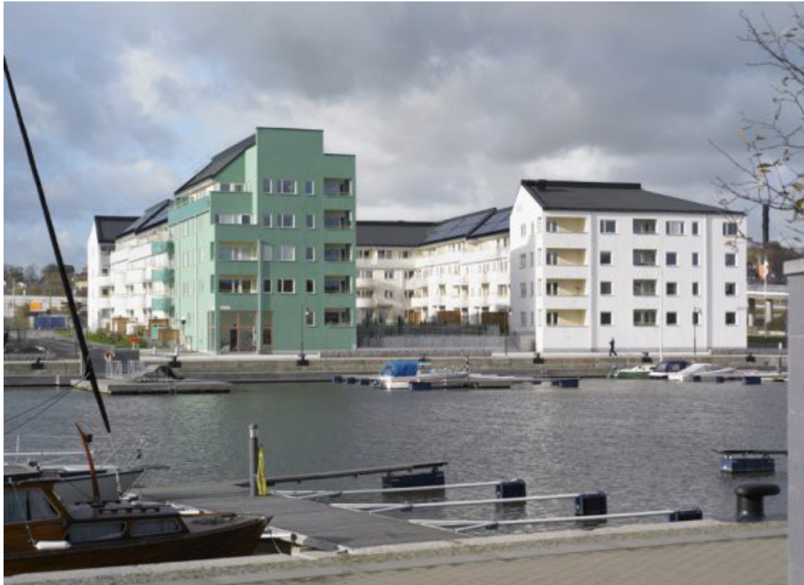
Hamnhuset – Passive House – Energy Efficient Building - Gothenburg
